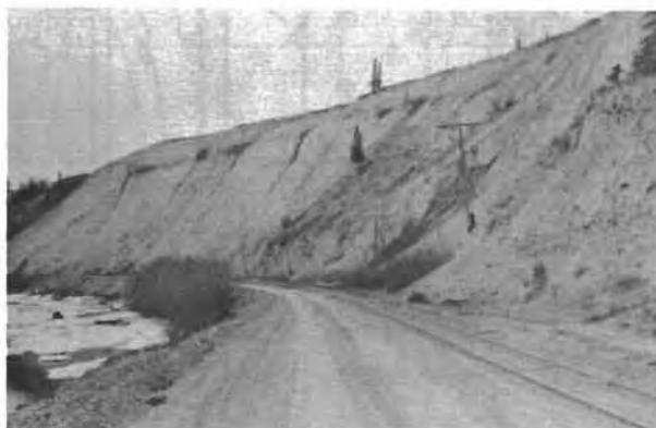
Figure 16. Steep, dry slope adjacent to railway south of Whitehorse, May 1957. Note occurrence of some gullying on face and also soil stratification on right side of photo (DBR photo BR 6772)
