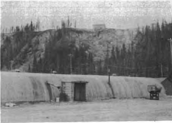
Figure 7. Sloughing on slope at DOT garage (at top of bank), May 1957 (DBR photo BR 6763)
